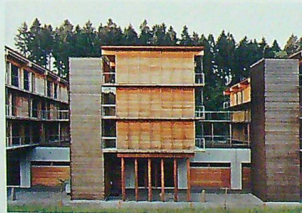
Şekil 6. Lyss Foresters College, cephede ahşap kullanımı (17). Figure 6. Lyss Foresters College, use of wood on the facade (17).
