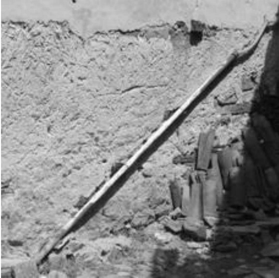
Figure 5. Unhealthy Sewage Pipe
